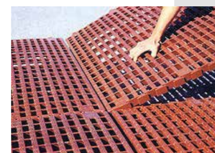
Detail of grid's assembly
